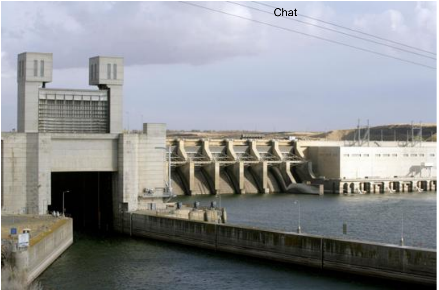
Ice Harbor Dam, one of four dams on the lower Snake River.
